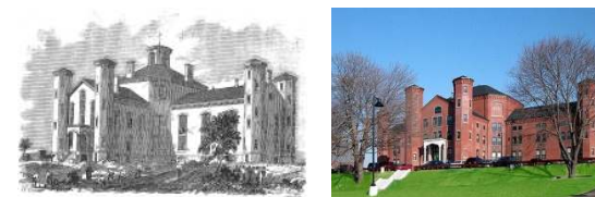
Figure 2. "The Castle" in South Portland. First the Reform School, now MMP Urology
